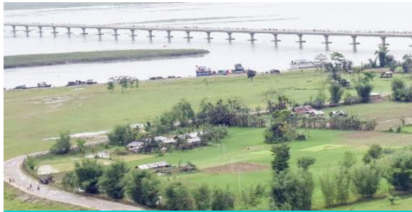
4 Lane Flyover at Mission Chairali, Tezpur, Assam
