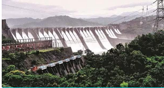
Lower Subansiri Hydro-electric Project, Arunachal Pradesh
