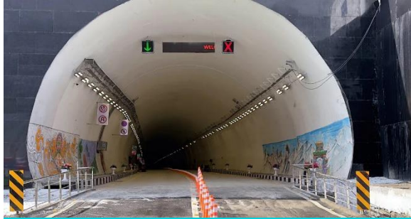
Sela Tunnel, Arunachal Pradesh
