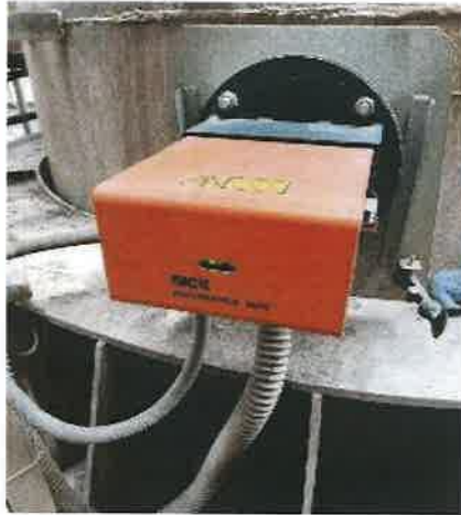
Sick Opacity meter in all stacks
