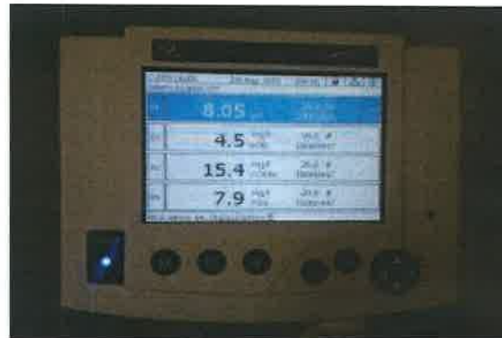
Online Monitoring at STP
