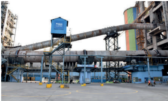
Cement kiln at Dalmia Bharat Limited's Rajgangpur plant in the state of Odisha in India.
