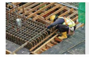
The shuttering should be strong enough to withstand the weight of the concrete, reinforcement of the steel, weight of the people involved in placing and compacting the concrete, impact loads due to the concrete placement, and vibrations from the vibrator.
