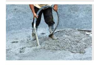
The freshly-prepared concrete may contain entrapped air and it should be removed by compaction through the process of vibration (with the help of needle or plate vibrators). Proper compaction of concrete is extremely important, as for every 1% void in the concrete, its strength reduces by 5%.
