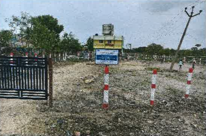
Fencing at Ottakovil PHC
