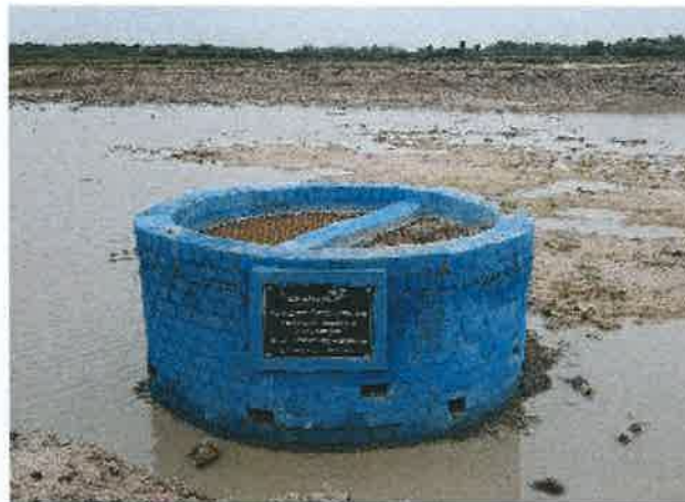
Bore well recharge pit at Eluppaiyur and Kamrajapuram
