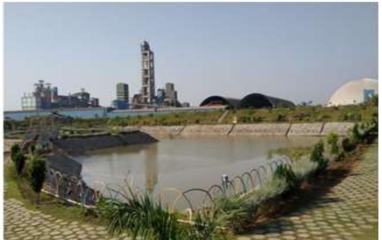
Plant Rain Water Harvesting Pond
