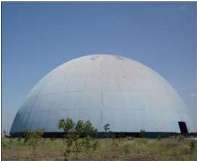
Lime Stone Storage Shed
