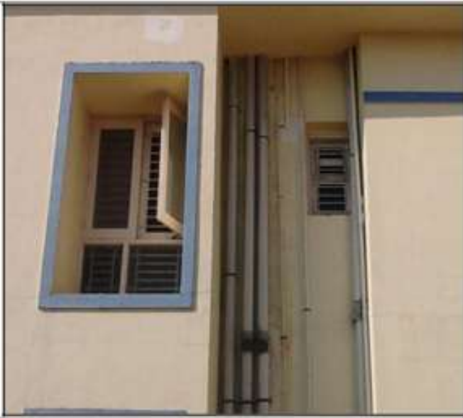
Rooftop Harvesting in Colony
