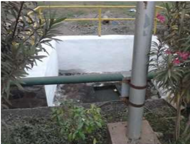
Drain Water Harvesting Pit
