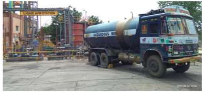
Mechanized system for unloading and feeding AFR weigh feeder and Rotary airlock. 5KL/Hour through calciner and 10KL/Hour through Kiln, Storage Capacity of 50KL Storage capacity of 100MT.
