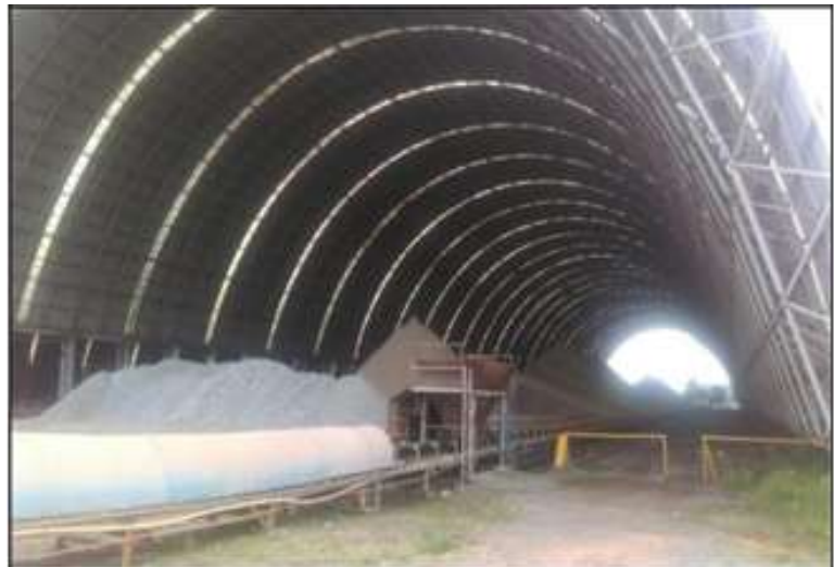
Coal & Additive yard
