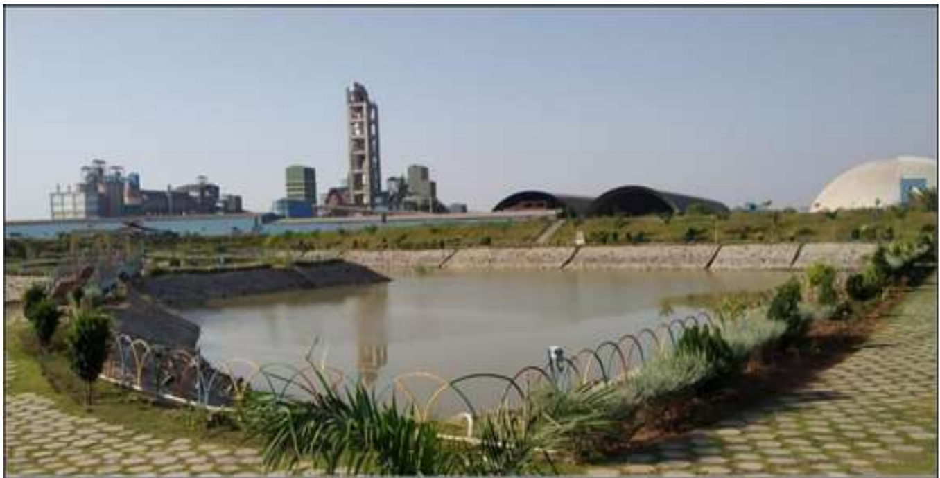
Plant inside Rain Water Harvesting Pond
