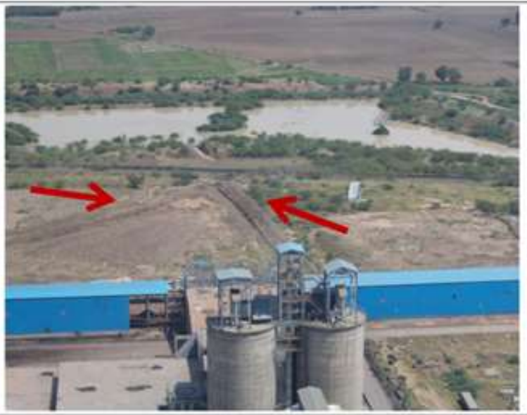
Storm Water Drains connected to Pond
