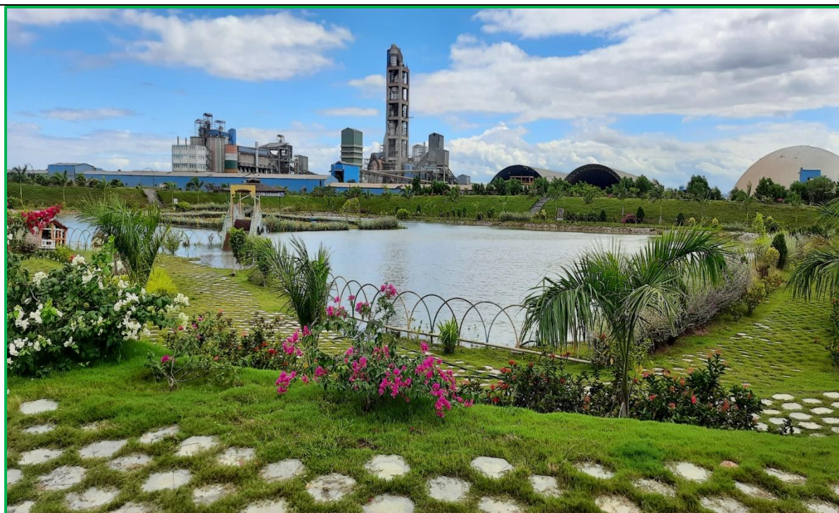
Rain Water Harvesting Pond at Plant
