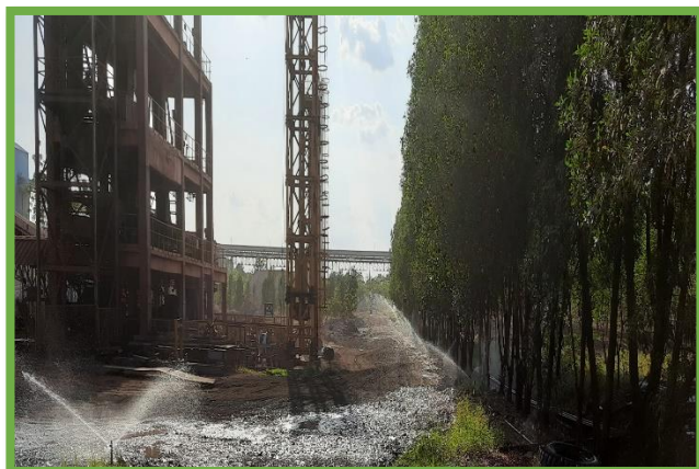
Water Sprinklers at RMH Area
