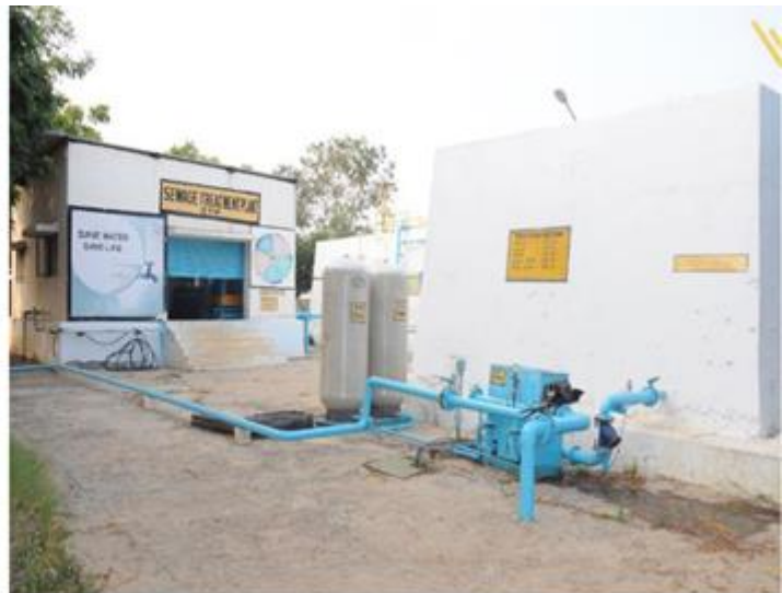
Sewage Treatment Plant
