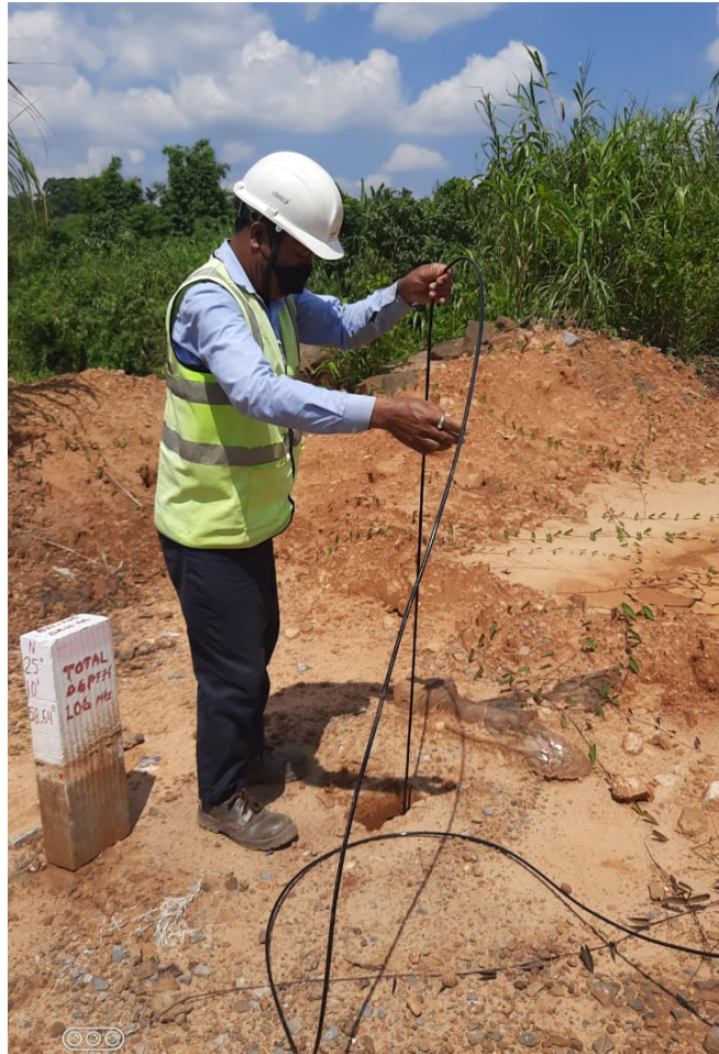
Fig. 22. Lowering of piezometer at the borehole#2 with depth of 106m bgl in the location 92^{\circ}21' 32.4''E - 25^{\circ}10' 58.62''N at the Umsoo Mootang mine in September, 2023.
