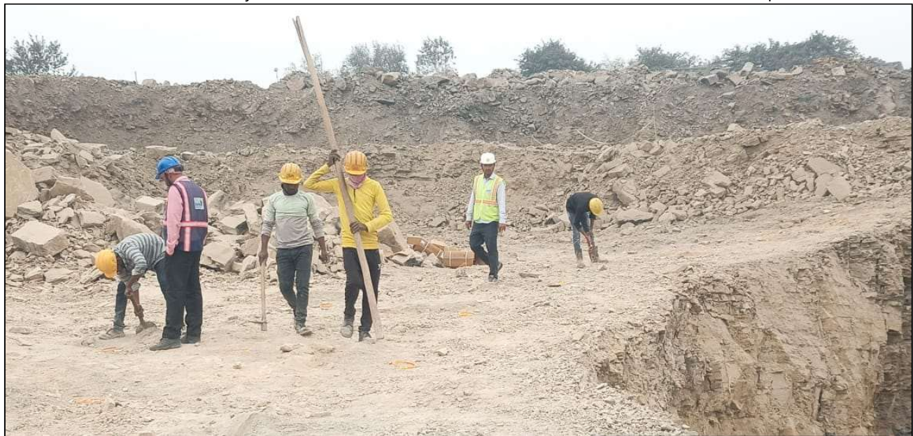
Figure-10: Stemming & Connection of TLD's in presence of technical Support team
