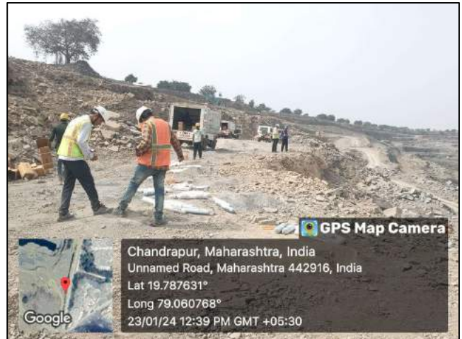
Figure-12: Measurement of drill hole parameters
